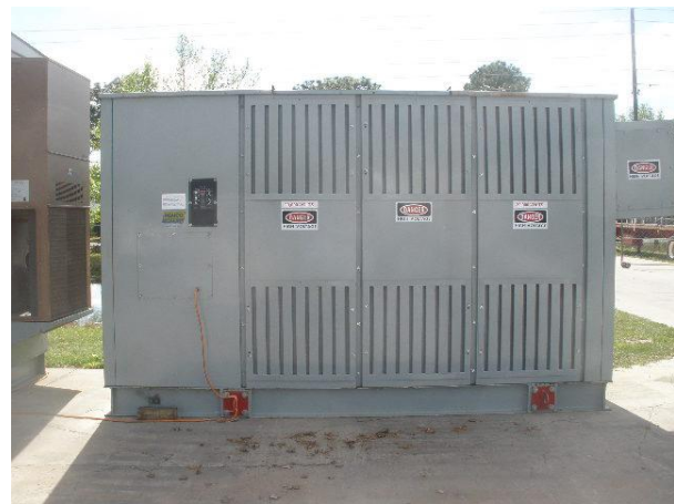
Above, a Basler Cutler Hammer ECS-2100 with the ECS-2100 Dry Type Transformer.
