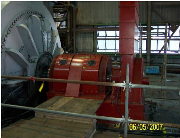
Above left, a 7200 amp collector assembly coupled to the generator and tied into our mobile exciter, on right the remote panel in the control room for full automatic operation.
