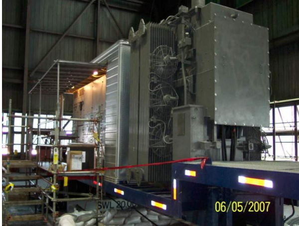
Mobile exciter and collector installed on an emergency rental in midwest region of US.
