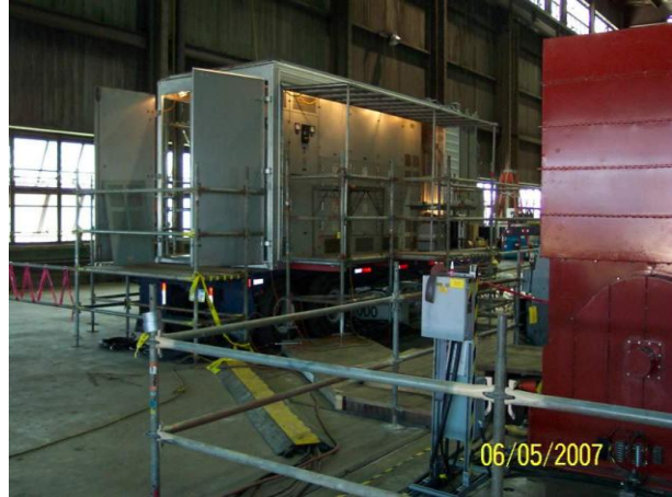
Mobile exciter and collector installed on an emergency rental in midwest region of US.
